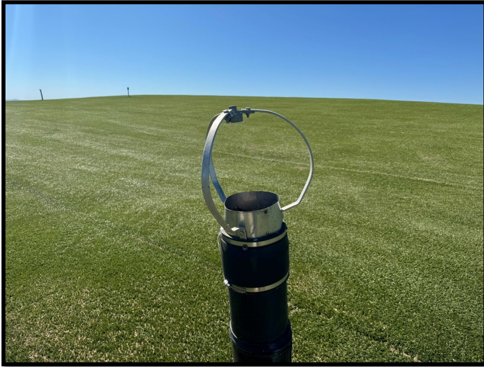
Photograph 19: View of damaged turbine vent near LCS-6 before repairs.
