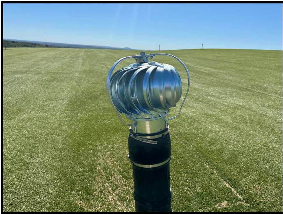
Photograph 20: View of turbine vent near LCS-6 after repairs.
