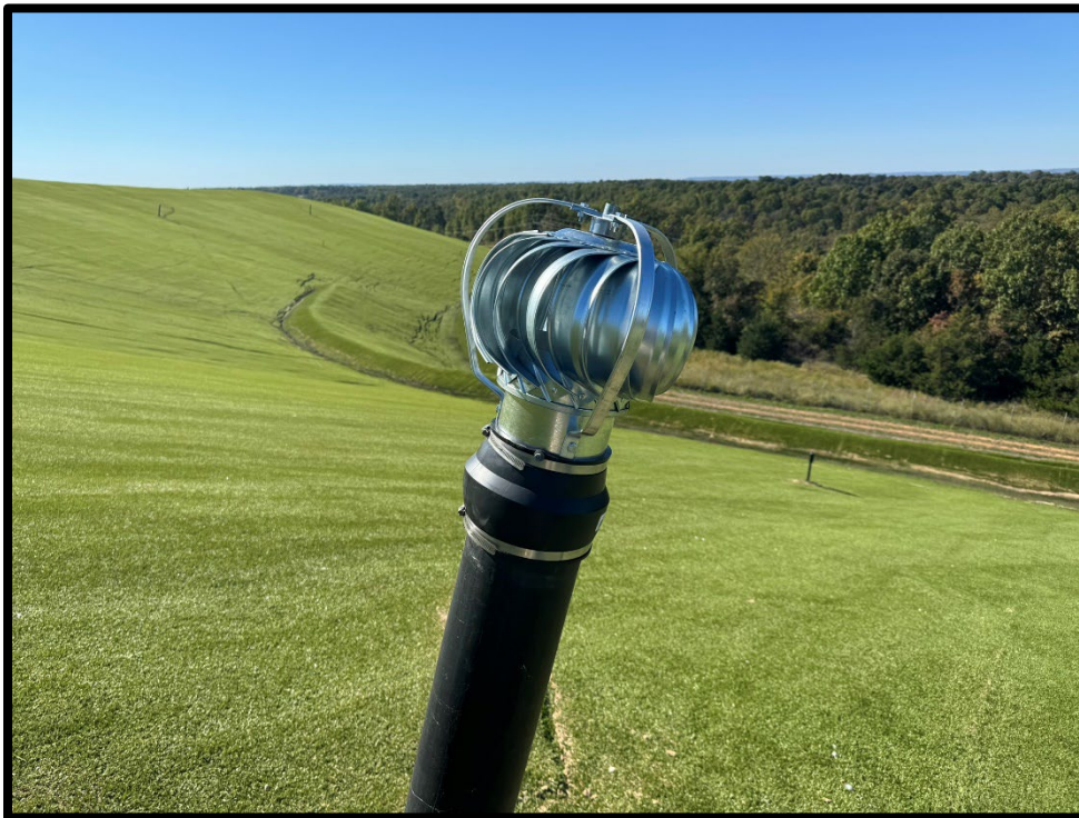
Photograph 18: View of turbine vent on north side of Area 1-2 after repairs.
