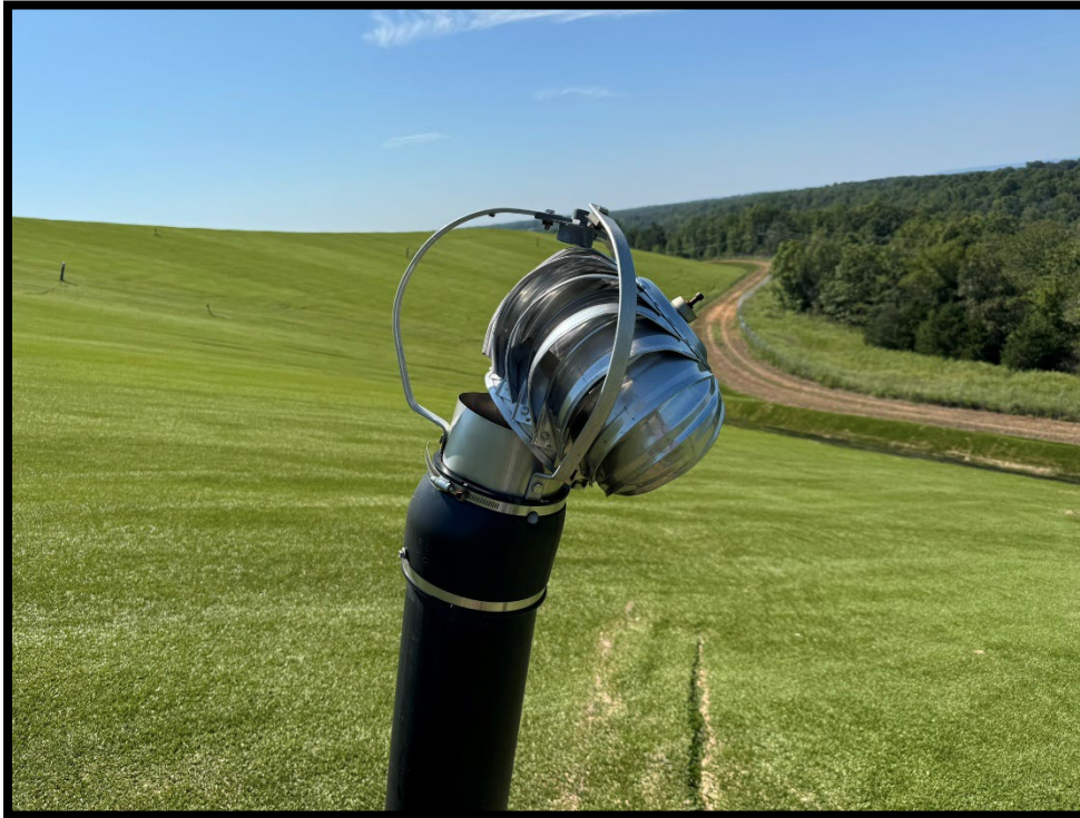
Photograph 17: View of damaged turbine vent on north side of Area 1-2 prior to repairs.
