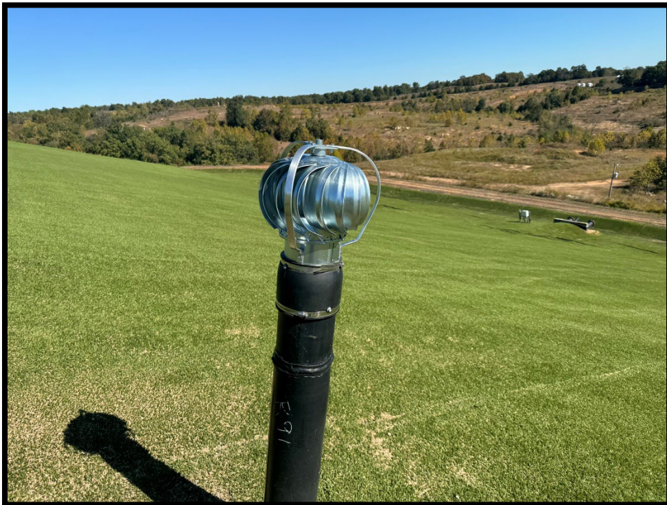
Photograph 22: View of turbine vent near LCS-8 after repairs.
